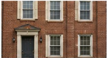
Brick rowhome masonry
