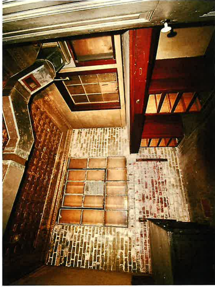
Warehouse 2nd floor space
